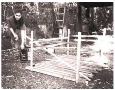
I put a lot of work into the supports because they are what give the stand strength. I sawed the ends of each support at angles so that they slid between the vertical bars that they were supporting.
