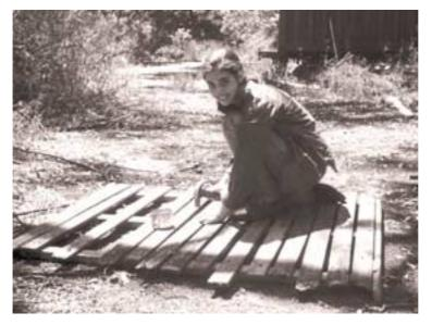
Once the floor was completed, I made the walls by nailing the wood into roughly 'H' shapes. I then began measuring and sawing the supports.
